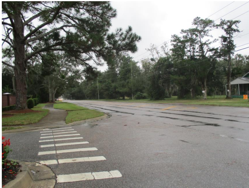
View of the Subject Property along Yellow Bluff Road.
